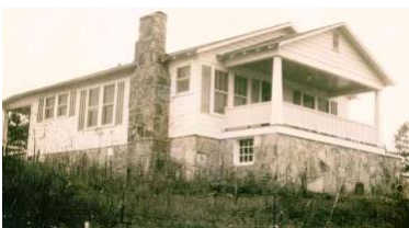
THE GLASSCOCK HOME VANDIVER ROAD
