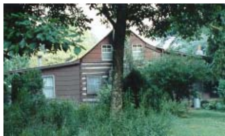
YOU CAN SEE THE ORIGINAL LOG HOUSE. THE AREA ON THE BACK (TO THE LEFT) EXTENDS ACROSS THE BACK OF THE HOUSE. THERE IS A BEDROOM ON EACH END WITH THE KITCHEN IN THE MIDDLE. THE FRONT PORCH WAS ADDED TO THE FRONT OF THE LOG HOUSE, BUT IS NOT VISIBLE DUE TO THE TREES.
