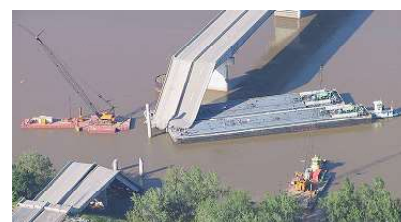
Collapsed I-40 Bridge, near Webbers Falls, Sequoyah County, OK -- May 31, 2002
