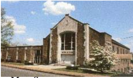
MAIN STREET CHURCH BUILDING 322 N. MAIN STREET
