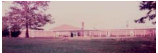
THE SCHOOL BUILDING AT NEW UNION
